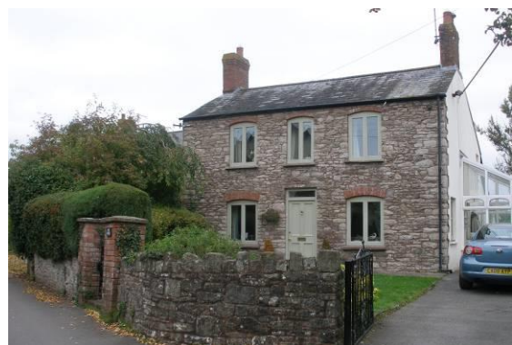
Figure 62 The Ferns. An attractive 19 th century cottage, standing behind original cast iron gates. Its red brick voussoirs contrast well with the rubble stone walls. The well-designed timber casement windows are probably replacements.
