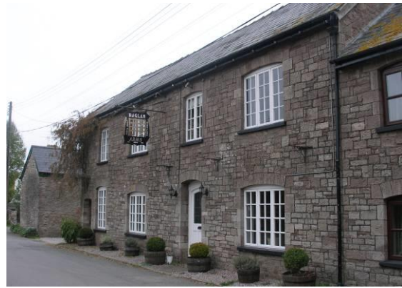
Figure 60 The Raglan Arms. The flush façade and regularity of fenestration is enhanced by the fine detailing of its stonework, especially in the ‘random’ coursing and dressings and well executed cambered stone window heads.
