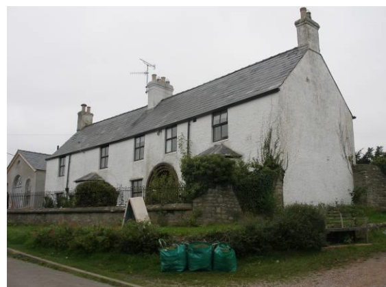
Figure 49 The former vicarage, a vernacular building, altered with Victorian and 20 th century additions.
