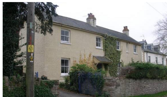
Figure 55 The Grange. A wider frontage, shallow depth type with original Victorian sash windows.
