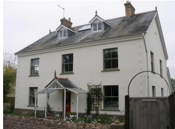
Figure 63 Holmer House. The simple symmetry of this substantial Edwardian house is enlivened by decorative bargeboards to the dormers and porch, the ornamental ridge tiles and finials and the patterned brickwork of the chimneys.
