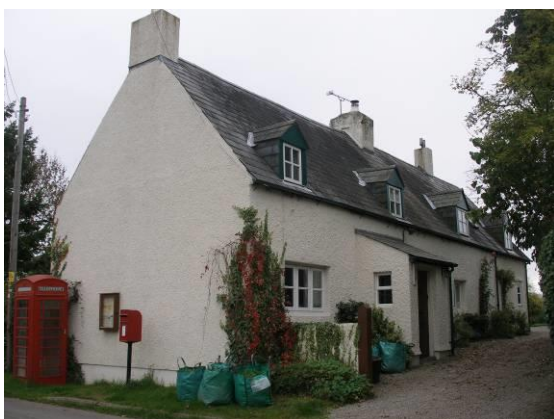
Figure 48 Orchard House. A vernacular cottage row set at right angles to the street. Typical features of this type of building are a long low profile, steep pitched roof, 1½ storey height, chimneys at the ridge and gable end and small casement windows.
