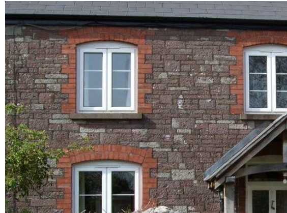
Figure 66 An example of snecked stone on Sycamore House
