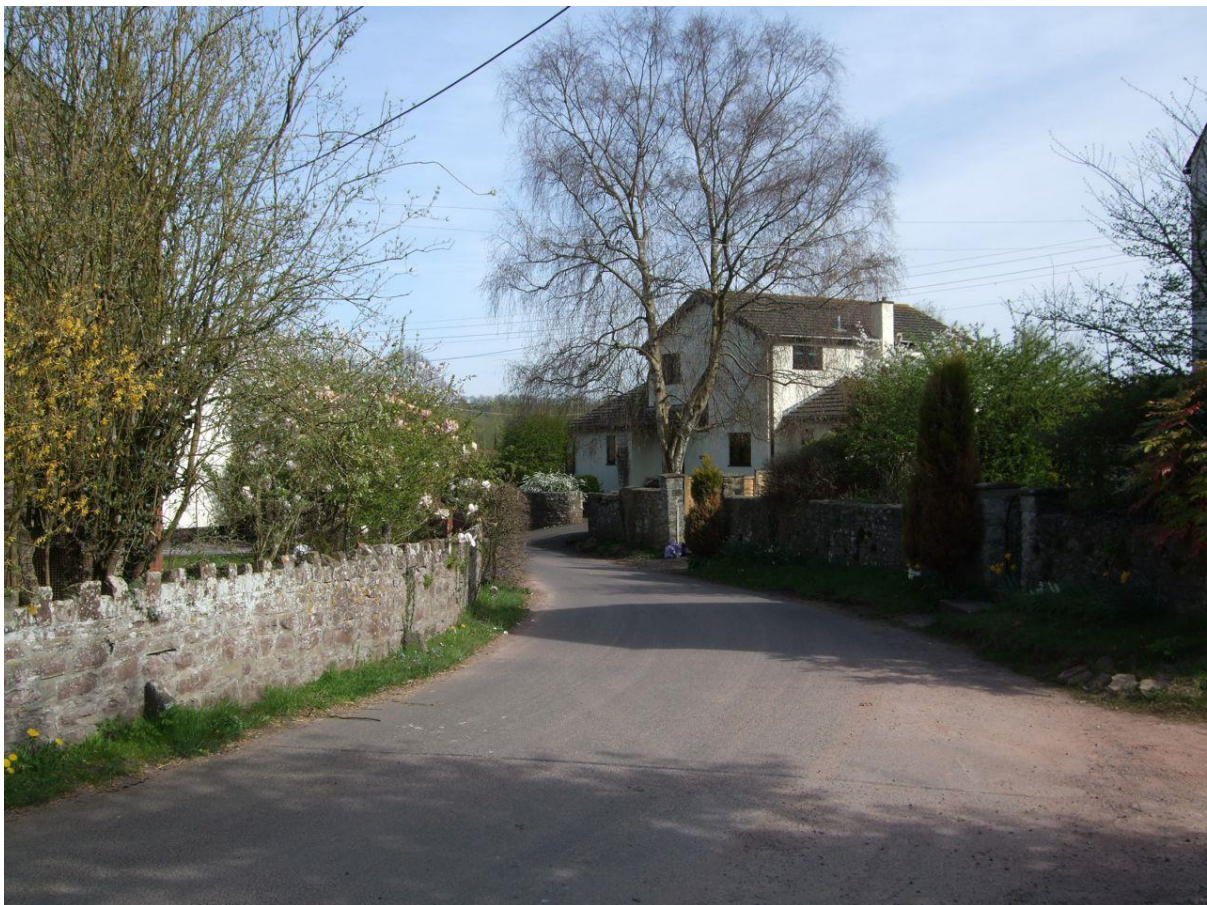
Figure 69 Examples of stone walls found in the village
