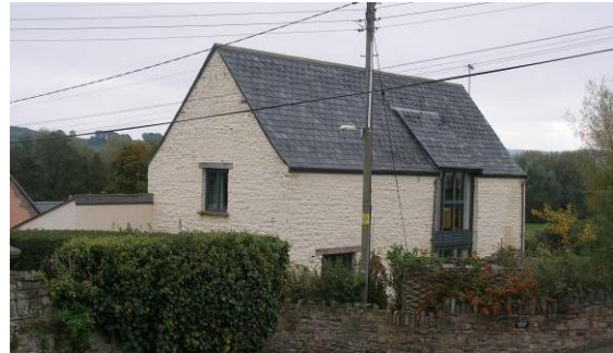
Figure 53 Willow Barn. This sensitively converted barn, part of the Church Farm/ Village Farm complex retains most of its original features.
