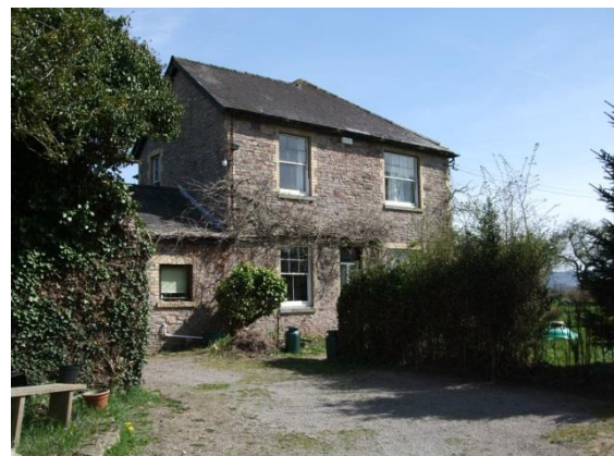
Figure 34 Historic sash windows survive at Oakfield
