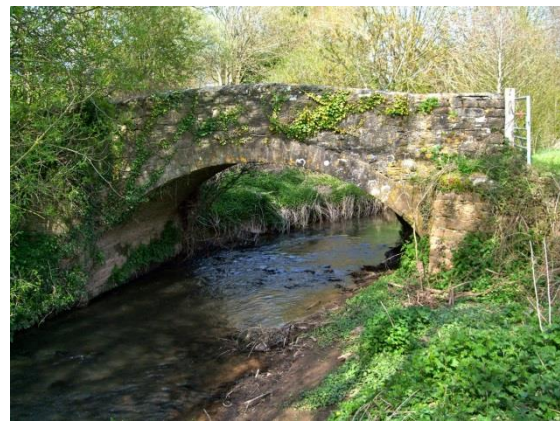
Figure 44 The stone arched bridge across the Olway Brook, now partially obscured by vegetation
