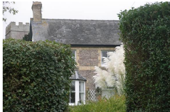
Figure 61 White Lodge. A well preserved example of a modest Victorian country house, with its sashes and bay windows retained in their original form. The ‘natural’ colour scheme of the purple-grey slates, the warm light grey stone, and the yellow-buff brick dressings and string course, highlighted by white painted glazing bars is extremely effective.
