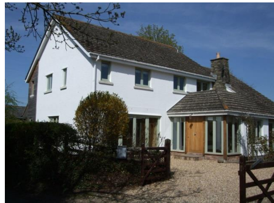
Figure 67 The rendered and weatherboarded Oakways
